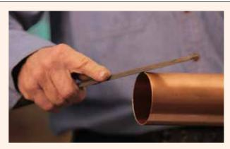
**2.** Carefully deburr and wipe clean the end of the tube internally and externally to minimise turbulence and pressure loss according to AS3500 and avoid damaging the O-ring.
