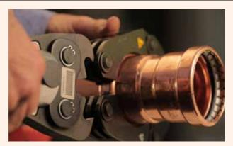
9. Open the ZB203 Adaptor Jaw by depressing the jaw levers and attach to the press collar so that the claws of the jaw grip around the pins of the press collar. Initiate the pressing job by pressing the start button. The pressing procedure should not be interrupted prematurely unless in an emergency by pressing the emergency stop button. The KemPress tool will flash if the fitting does not press correctly.
