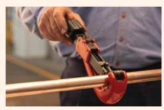
1. Cut copper tube to length using a pipe cutter.
