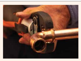
7. Check the fitting outer edge still lines up with the marking. Open the pressing jaw and close it around the fitting so the raised bump in the fitting rests inside the groove of the pressing jaw. Ensure the jaw is engaged square with the fitting and not on an angle.
