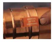
For DN65-100 fittings, remove the KemPress® label to indicate completion of the press.
