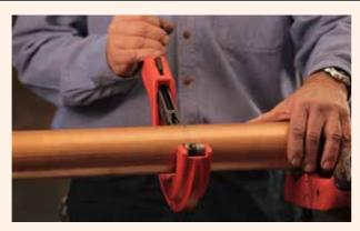
**1.** Cut copper tube to length using a pipe cutter or fine tooth saw and ensure the pipe is cut square.
