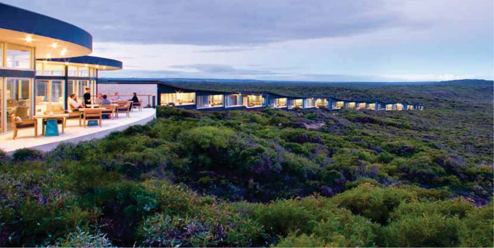
Rheem Commercial Heat Pumps provide hot water to Southern Ocean Lodge — Kangaroo Island, SA
